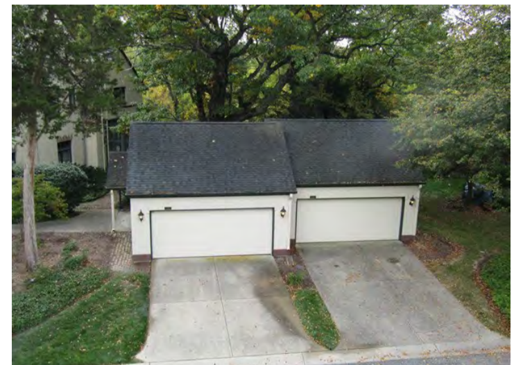
detached garage serving mansion
